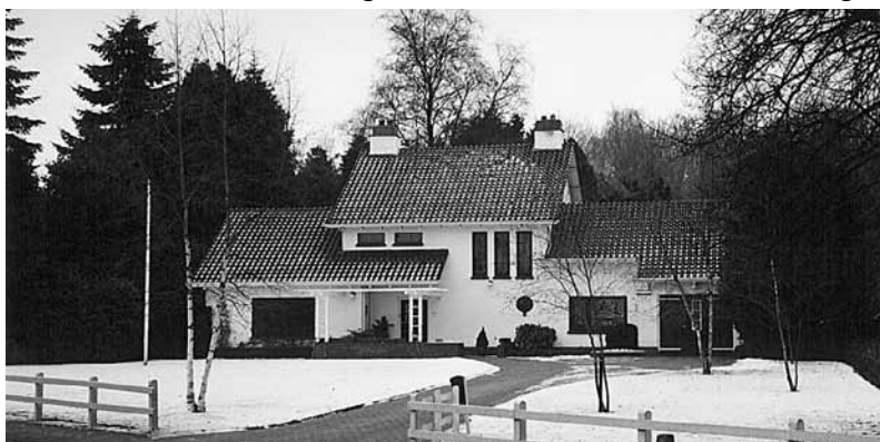
Barchemseweg 56 (1935, architect G.J. Postel)
